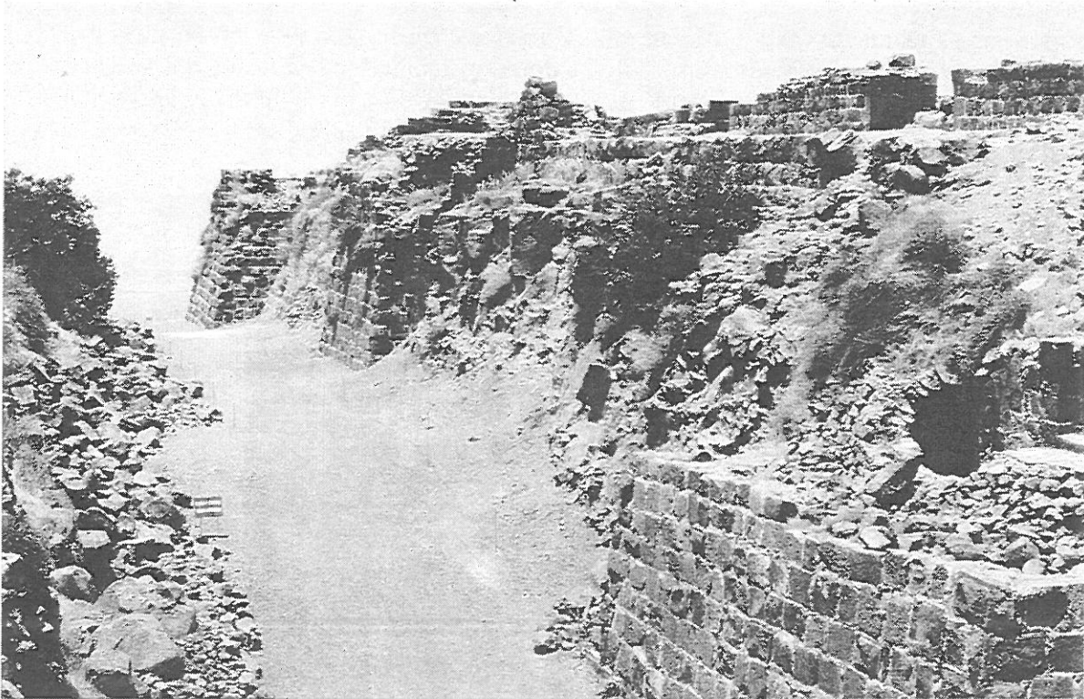
11. Belvoir. South-west corner.
