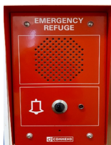
Commend refuge communications intercom
